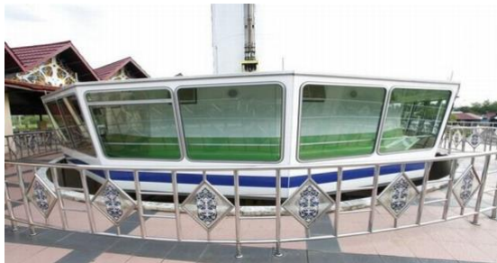
Gambar 13 Wahana Tower Pulau Kumala
