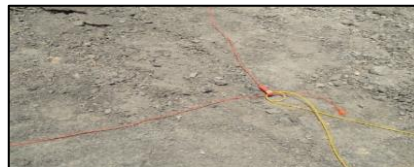
Gambar 4.22 Proses tie up
