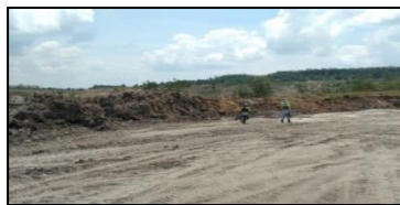
Gambar 4.25 Penarikan Lead Wire kearah Shelter
