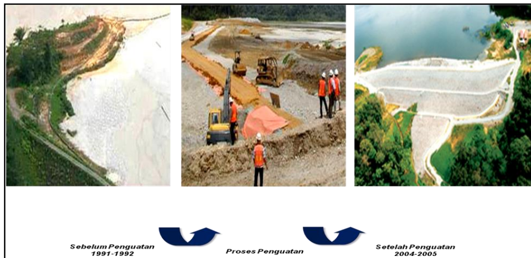
Gambar Penguatan DAM Namuk PT. KEM
